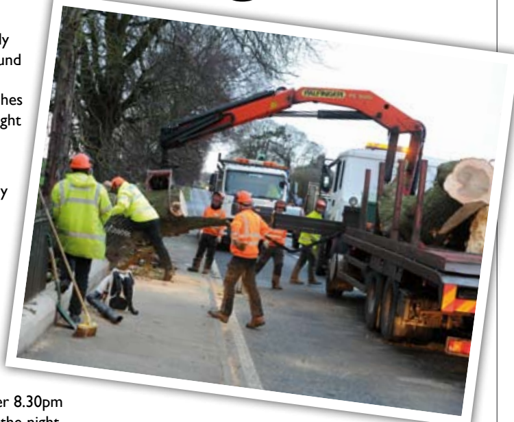
WORKING AROUND THE CLOCK: Teams remove a fallen tree in South Cave Images courtesy of Hull Daily Mail
